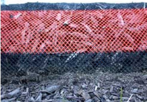
A 3-Dimensional Compost Filtration Matrix traps silt inside the socks
