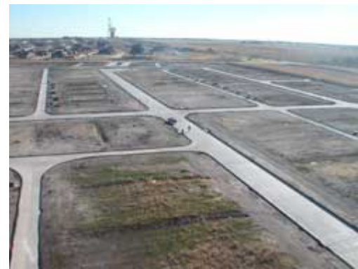
Keeps the Entire Site in Phase II Compliance
